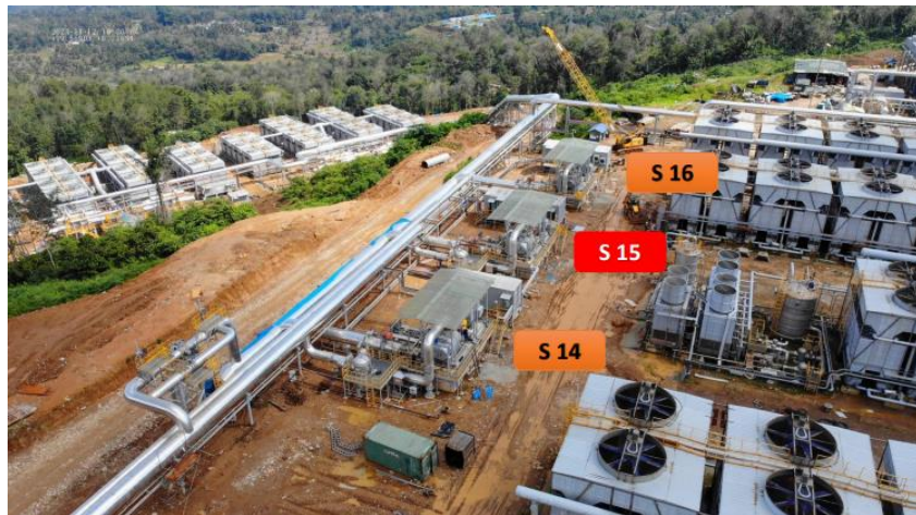
Gambar 3. 14. Steam Expander Modul S-14 s.d. S-16 PLTP Sorik Marapi Unit 4 (total 39,6 MW)
